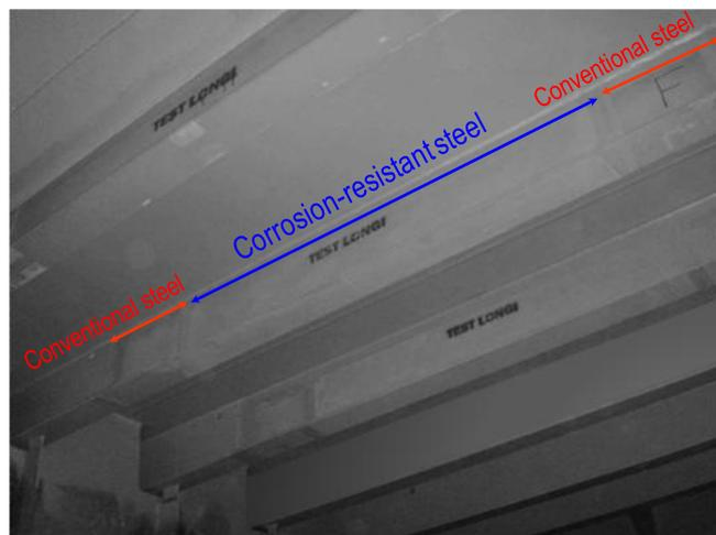
Fig. 11: Appearance of a test longitudinal for a water ballast tank
