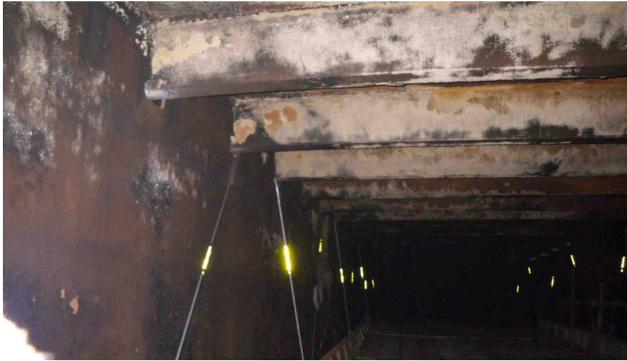
Fig.5 Opposite Side of Web - Staging Wire Shown
