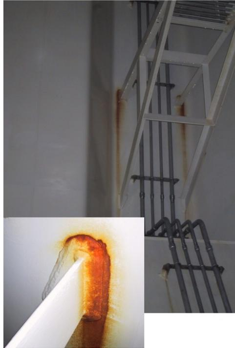
**Figure 9 Accelerated corrosion in way of attachment points**
