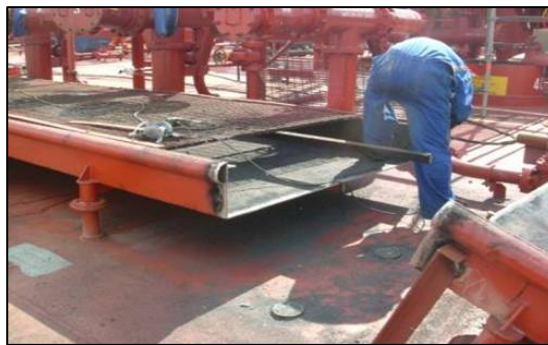
Drip tray being modified from continuous to several separate sections
