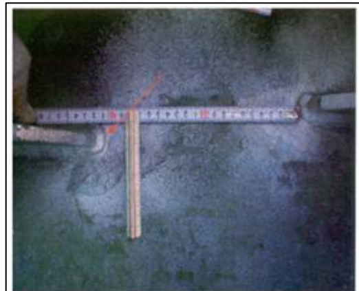
Figure 35 Misalignment Brackets of Vent Riser Pipe Support
