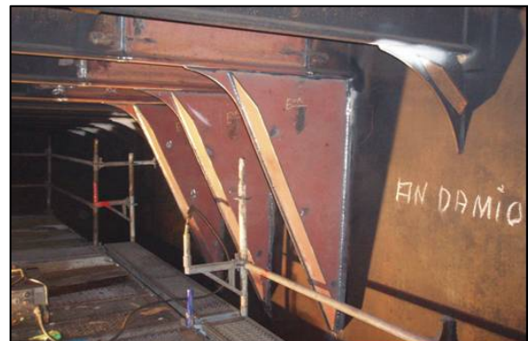
Local repairs / alterations in way of local underdeck girders
