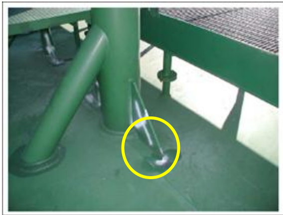
Cracks at the pipe support bracket connection to main deck toe
