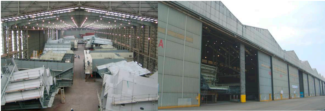
Fig.1 Weather controlled indoor blasting & painting facility
