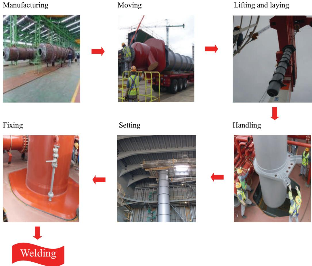
Fig. 10 Installation sequence of KVOC
