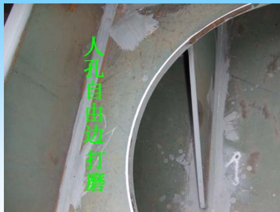
Fig.6 Sample plates of structure treatment
