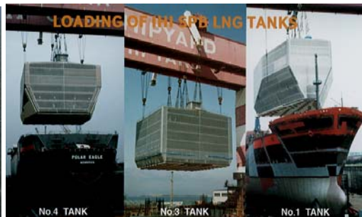
Loading of SPB tanks
