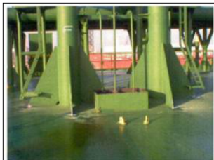
Figure 34 Deck Cracks: TWO Bracket Toes of Vent Riser Pipe Support
