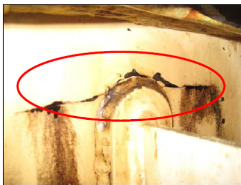
Crack in way of ladder lug doubler – connected to unsupported plate of oil tank. Vibration induced crack.
