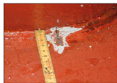
Close-up showing crack in deck plating.
