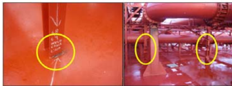
Crack i.w.o fillet welding i.w.o pipe support connection to upper deck.
