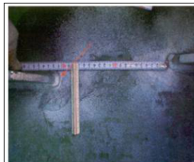
Figure 35 Misalignment Brackets of Vent Riser Pipe Support
